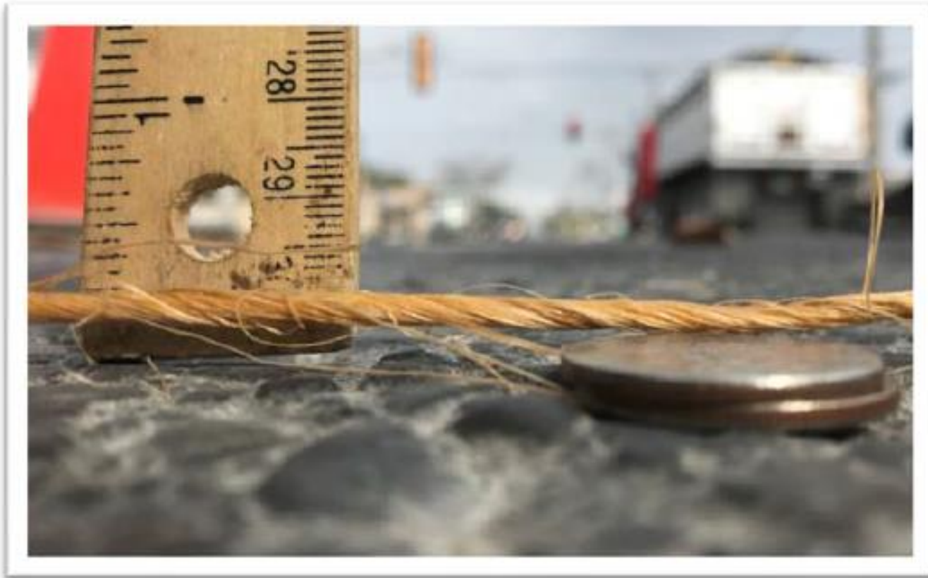
Rut Depth String Line, Williams St. Intersection
